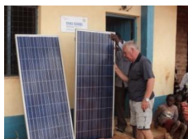
Eriks School - elektrifiering
